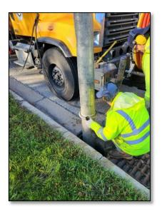
While manual cleaning with hand tools is sometimes necessary, vacuum trucks are the most commonly used type of catch basin cleaning equipment. They use a powerful vacuum to remove debris trapped by the basin. Two-man crews are usually required when using vacuum trucks. Vacuum trucks can also be used to clean stormwater pipes and other drainage structures. A storm sewer cleaning program is commonly implemented along with catch basin cleaning.
