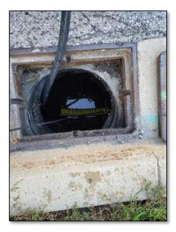
The most commonly used equipment for cleaning storm sewers is a jetter/vacuum truck. Jetter/vacuum trucks apply pressurized water to free and remove sediment and debris. Other types of equipment that can be used to clean storm sewers include hand tools for manual removal of smaller amounts of sediment and debris, and bucket loaders to remove larger amounts.
